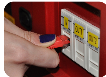
Figure 10 Connecting a network cable
